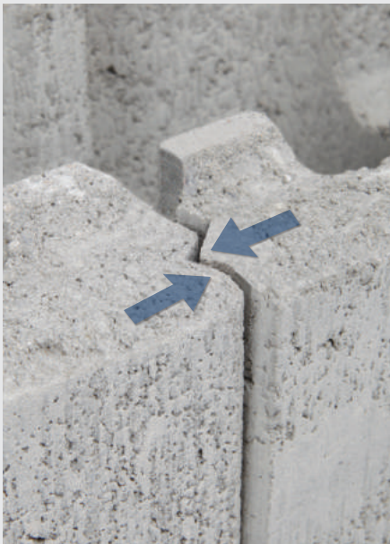
Interlocking tongue and groove joints
