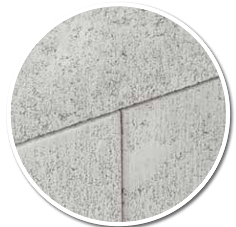
Clean wall with shadow lines
