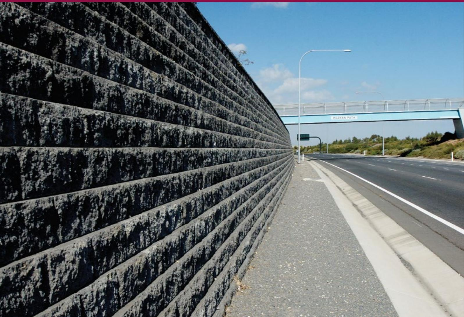
The designs provided in this brochure are for gravity retaining wall systems designed in accordance with the requirements of AS4678 “Earth-retaining Structures”.
