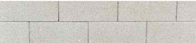
Versastone® features an architecturally inspired shotblast surface texture which exposes the natural aggregate stones in each block. This premium, dry stack, interlocking retaining wall system is available in a range of modern colours adding depth, dimension and enviable aesthetics to your project.
