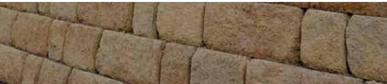
The Diamond Pro Stone Cut™ retaining wall system is a multi piece retaining wall system that recreates the random, distressed appearance of a natural rock face providing the opportunity to build very tall, durable, commercial retaining walls that effortlessly compliment any natural environment. The addition of the Anchor Wall® rear lip system ensures uniform setback, proven grid connections and easy installation.
