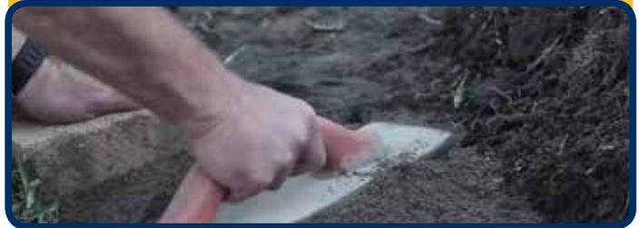
The fun part! Start at one end and place blocks onto the screeded sand and cement mix. Using a rubber mallet, gently tap the blocks into position and using your spirit level, check that each block is level with the one before it, side to side and front to back.
