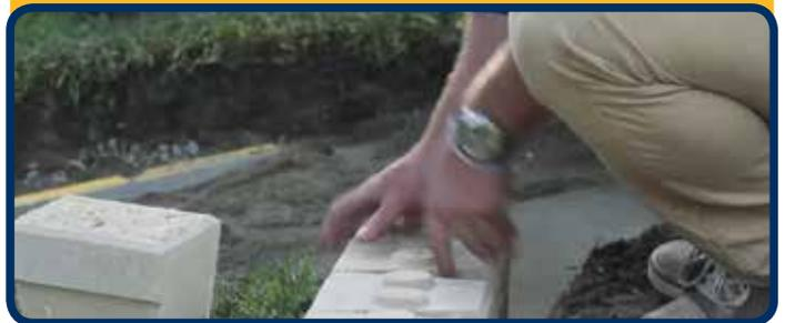
The job is almost done! Using a suitable landscape grade outdoor adhesive (such as landscape liquid nails) place 4 'blobs' of adhesive on the top of each block on your top course. Once you have done this, firmly place the capping unit into place on top of the glue.
