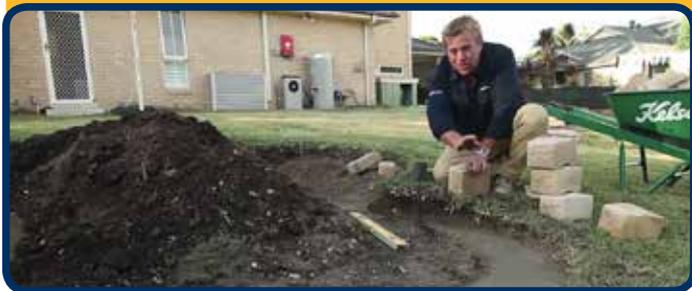
You can continue laying blocks by simply stacking them on top of one another – just like using children's blocks! Make sure you have a small hand broom to sweep dirt and debris off the top of the course below to ensure your laying blocks on a nice flat surface.
