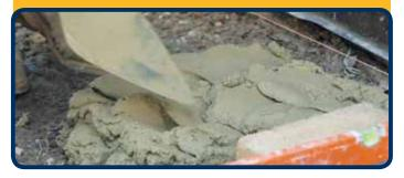
Prepare a sand and cement mix at a 4:1 ratio in a wheelbarrow. Be sure to mix the cement through the sand thoroughly while dry so you have a nice blend throughout. Add some water and mix until a thick, mud like consistency is achieved.
