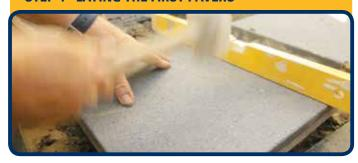
Place the first pavers on the sand and cement mix and wiggle over to string line but do not touch it. Check the level across the paver and then move on.
