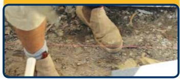
Make sure you set up a very accurate string line. Ensure the string line is level so all the pavers you lay are level.
