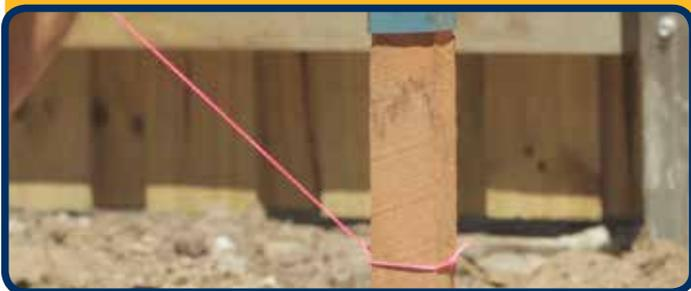
Mark out the location of your garden edge. Set up a string line and mark the area to be excavated with a spray on marking paint. If your edge curves, you can use rope or even the garden hose to mark over.
