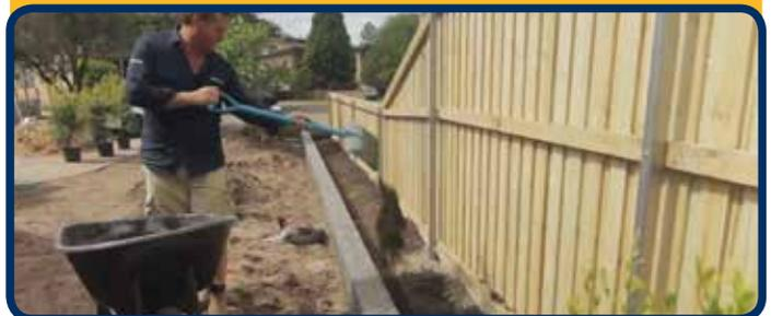
After allowing suitable time for the glue and caps to dry, you can begin bringing in the soils for your garden bed. Aim to fill behind the edge to approximately half way up your capping unit. A handy tip is to firstly fill behind your edge to about half way and then place your plants, flowers and trees before then filling the rest of the way with soil - this will save you digging new holes later!
