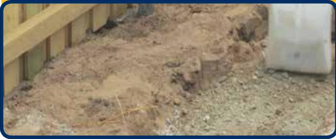
Spread road base through the trench and work towards an even surface. Then, with a plate compactor (wacker-packer), go over the area two to three times to ensure road base is compact and firm.
