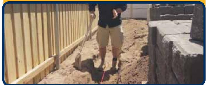
With a spade, excavate the marked area to approx 200mm in depth which allows for 100mm of road base, 30mm of sand and a portion of the block for your first course to be below ground level. Remove any rocks, root or debris and compact the base of the trench.
