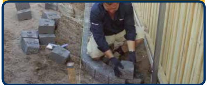
Once the first course is complete, subsequent courses are simply stacked on top of the blocks below using a stretcher bond pattern. Be sure to sweep off any loose material sitting on top of the blocks that may affect the placement of the next course and continue to check the wall is level as you go.
