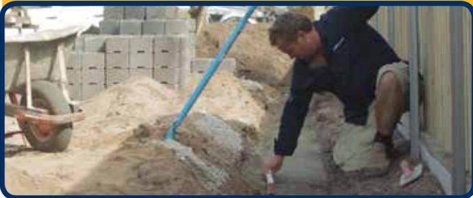
You can now begin laying the blocks. Set up a string line along the length of the wall to ensure all blocks remain flush and straight. Place blocks on the sand, check level and tap into place with a rubber mallet. Continue laying blocks tightly next to each other through the length of your wall.
