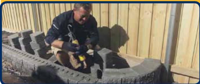
Once you have finished laying your garden edge blocks, you need to secure the capping units to the top course of the garden edge. Sweep the top of each block first to remove dirt and rubble. Then with a landscape adhesive in a caulking gun, place 'blobs' of glue on the front and rear of your top course and firmly place the speciality capping unit. Use a rubber mallet to tap down and check level in both directions.
